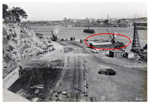
**Figure 2.5** Dorman Long Workshops site preparation, 18 March 1925. The construction of the Dorman Long Wharf can be seen on the right (circled in red). (Source: Luna Park Sydney Archives, 2015, from original held by State Records NSW, with GML overlay)
